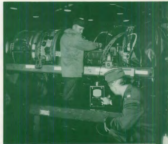
CMS William R. Morgart, presently at Luke AFB, inspects J-71 second stage blades using an ultrasonoscope. Insets show scope picture with center blip indicating cracked blade, and X-ray photo of the same blade.
